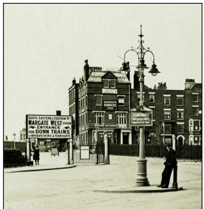
Station Road c. 1905 (note the ornamental gas-lamp and the eye-catching station-entrance sign) Courtesy of Anthony Lee
