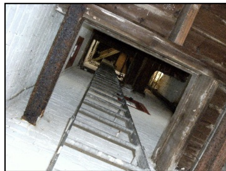
The metal ladder affixed to the wall inside the Clock Tower allowing access to the top of the building. Note the single stained-glass window to the right of the ladder
