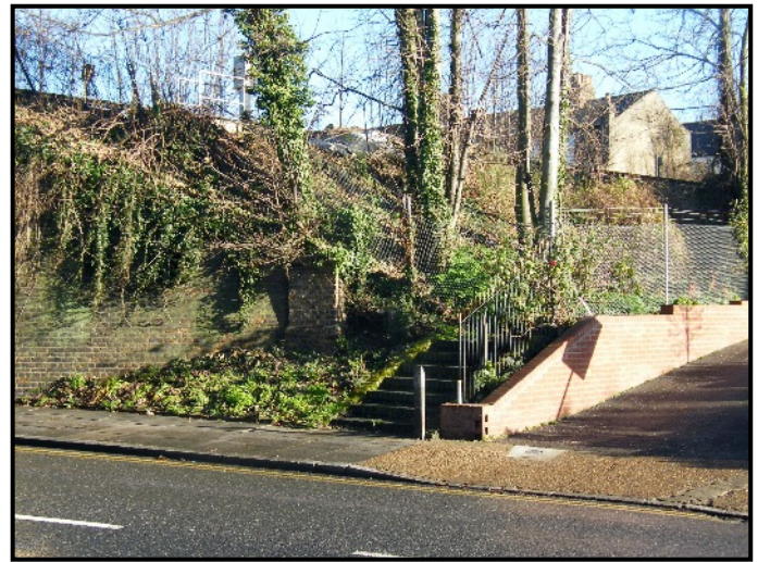
The flight of steps on the south side of the bridge over Ramsgate Road. Note the lengths of railway line being utilised as hand-posts. Another flight of steps complete with railway-line hand-posts can be seen on the north side of the bridge
