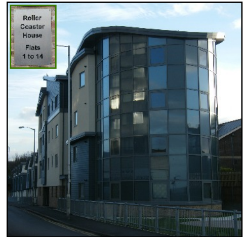
Roller Coaster House and associated housing, All Saints Avenue, Margate. Development by Town & Country Housing Group
